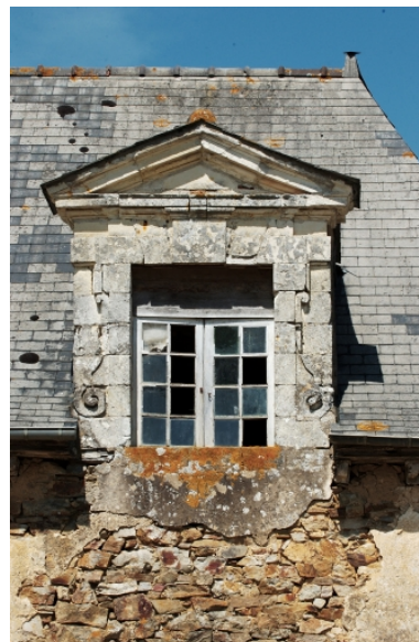
Lucarne en tuffeau Phot. Norbert Lambart IVR53_20053502025NUCA
