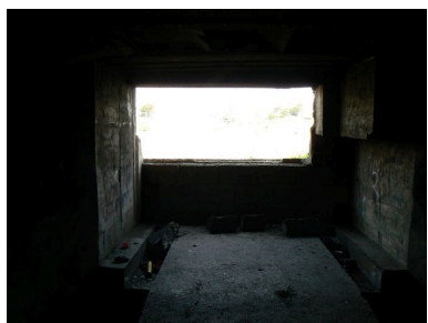
Embrasure de la casemate Phot. Julien Amghar IVR53_20082908632NUCA
