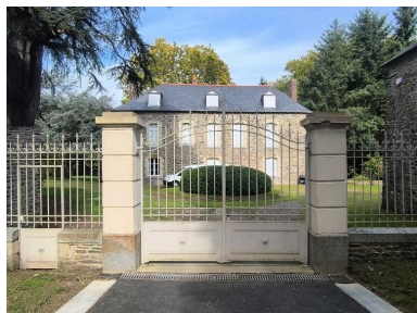
Manoir de la Retenue Phot. Annaig Point Mazzocchi IVR53_20263520041NUCA
