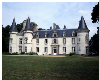
Elévation sud Phot. Guy Artur, Phot. Norbert Lambart IVR53_19935601811XA
