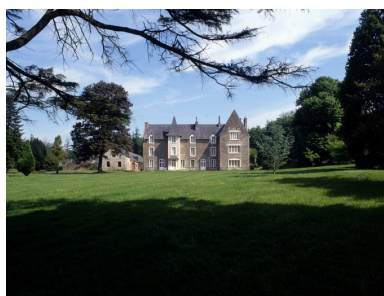
Elévation nord Phot. Guy Artur, Phot. Norbert Lambart IVR53_19935601810XA
