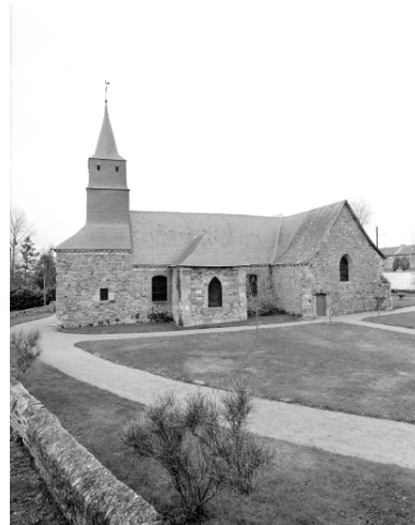
Élévation Sud Phot. Guy Artur, Phot. Norbert Lambart IVR53_19943500728X
