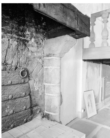
Cheminée, profil. Phot. François Dagorn IVR53_19785600564X
