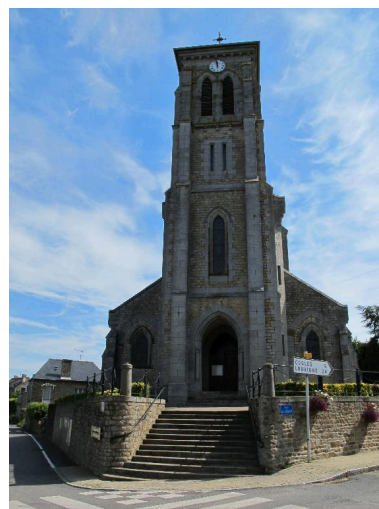
Façade principale Phot. Stéphanie Bardel IVR53_20133518048NUCA
