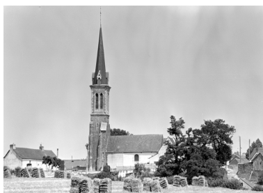
Vue de situation sud. Phot. Guy Artur, Phot. Norbert Lambart IVR53_19843500347X
