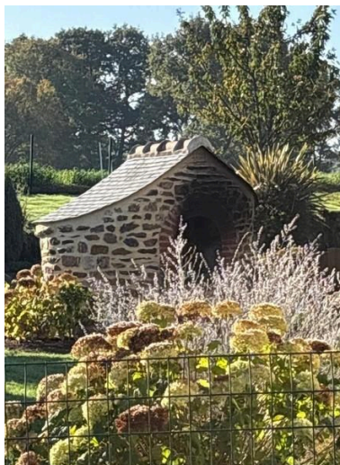
Four 1 l'Auseraie Phot. Annaig IVR53_20253531442NUCA
