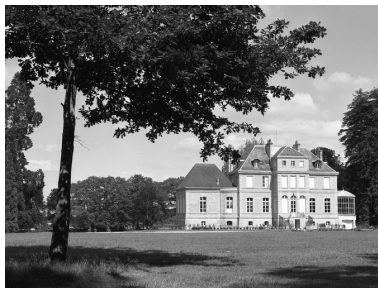
Elévation ouest. Phot. Norbert Lambart IVR53_19815600814X
