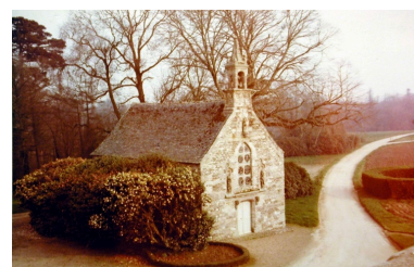
Chapelle (C.R.M.H. Bretagne) Phot. Elise Lauranceau IVR53_20033517763NUCA
