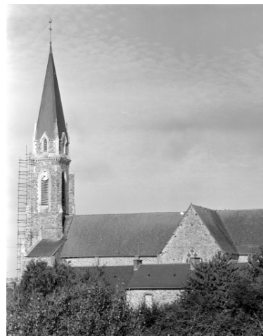
Elévation sud, clocher Phot. Guy Artur, Phot. Norbert Lambart IVR53_19943501388X
