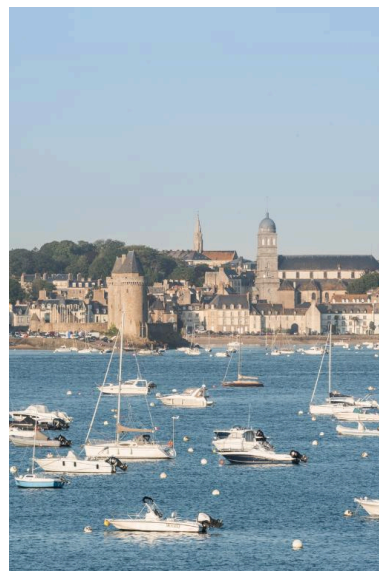
Vue de situation Phot. Charlotte Barraud IVR53_20203500500NUCA
