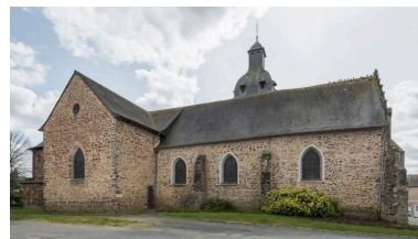
Elévation nord Phot. Delia Gaulin-Crespel IVR53_20183500133NUCA
