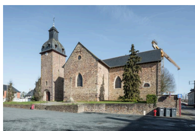
Elévation sud Phot. Delia Gaulin-Crespel IVR53_20183500105NUCA
