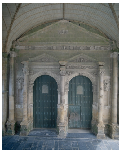
Porche ouest, porte principale Phot. Guy Artur, Phot. Norbert Lambart IVR53_19953500331XA
