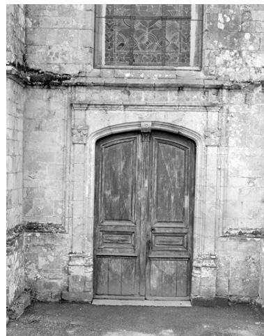
Façade nord, portail Phot. Guy Artur, Phot. Norbert Lambart IVR53_19943501494X
