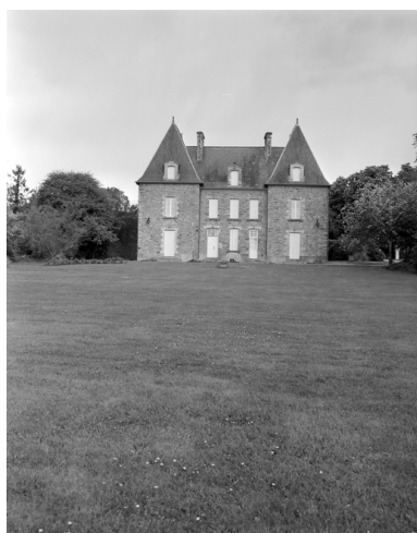
Élévation sud Phot. Guy Artur, Phot. Norbert Lambart IVR53_19963500873X
