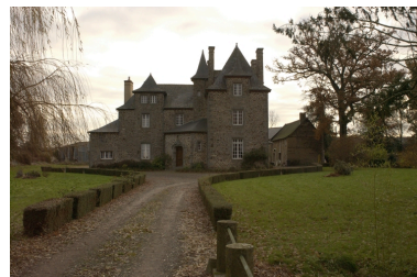
Façade ouest Phot. Norbert Lambart IVR53_20053503486NUCA
