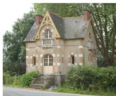
Conciergerie Phot. Norbert Lambart IVR53_20023503112NUCA
