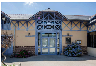
Phot. Anne Bonnafous IVR53_20193500857NUCA
