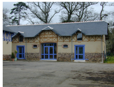
Communs Phot. Véronique Orain IVR53_20023512489NUCA
