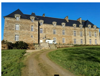
Façade sud Phot. Flavie Dupont IVR53_20252210095NUCA
