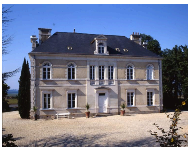
Élévation sud. Phot. Guy Artur, Phot. Norbert Lambart IVR53_19935601907XA
