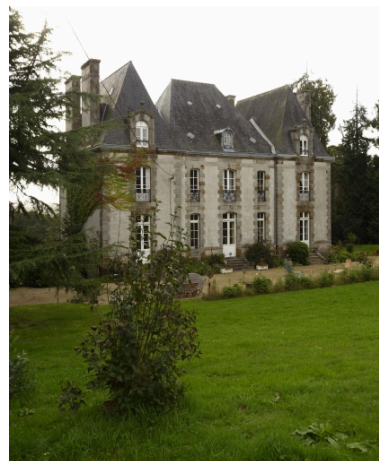
Elévation nord Phot. Norbert Lambart IVR53_20113503393NUCA
