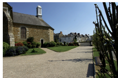
Vue partielle Phot. Norbert Lambart IVR53_20063500887NUCA
