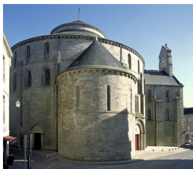
Elévation nord Phot. Bernard Bègne IVR53_20022900509XA
