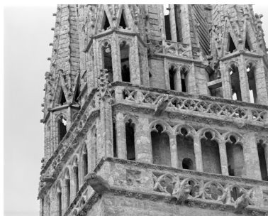
Clocher, galerie Phot. Lanvéoc-Poulmic IVR53_19802900475X
