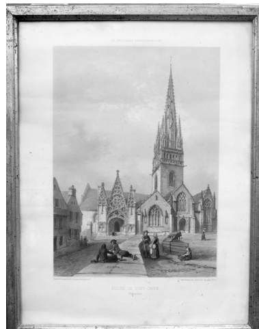
Elévation sud. Gravure ancienne. Coll. Gargadenec Phot. Guy Artur, Phot. Norbert Lambart IVR53_19832901104X
