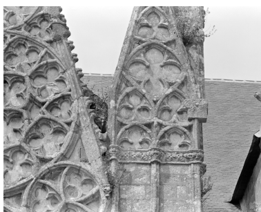
Porche sud, pinnacle droit Phot. Lanvéoc-Poulmic IVR53_19802900470X
