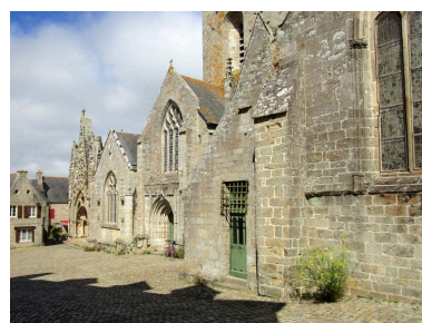
Elévation sud. (2022) Phot. Fabien Serre IVR53_20222906151NUCA
