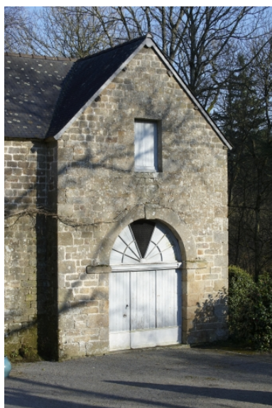
Ecurie, aile sud. Phot. Rozenn Turni IVR53_20113500541NUCA
