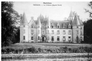
Façade nord Phot. Elise Lauranceau IVR53_20045606212NUCB
