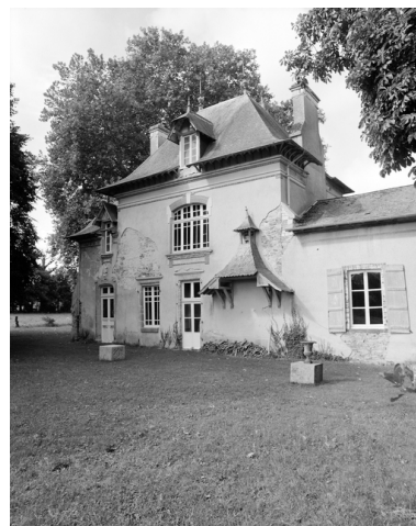
Vue générale est. Phot. Guy Artur, Phot. Norbert Lambart IVR53_19873500294X
