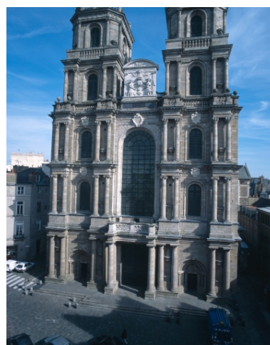
Élévation principale Phot. Guy Artur IVR53_20023501879XA
