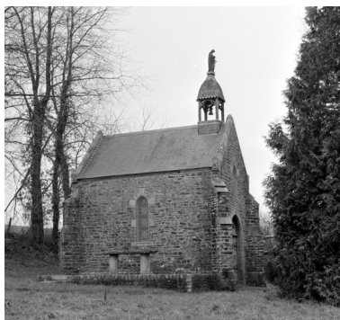
Elévation nord. Phot. Guy Artur, Phot. Norbert Lambart IVR53_19933500126X
