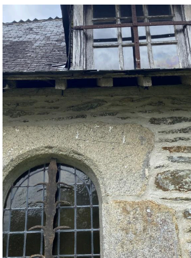
Date, élévation sud Phot. Baptiste Oligo IVR53_20265610397NUCA
