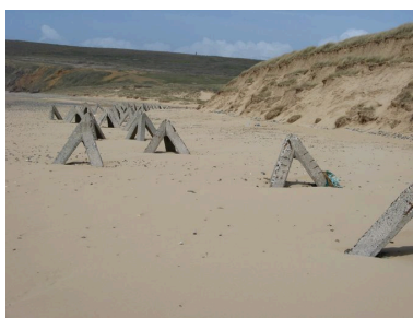
Obstacles de plage Phot. Guillaume Marie IVR53_20082908317NUCA
