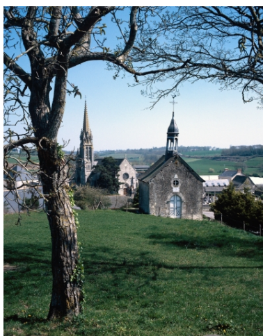
Vue de situation. Phot. Guy Artur, Phot. Norbert Lambart IVR53_19973500757XA
