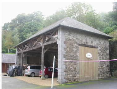
Remise Phot. Sabrina Dalibard IVR53_20063513820NUCA
