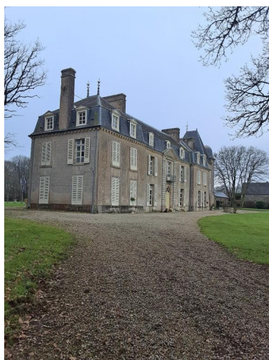
Façade sud Phot. Flavie Dupont IVR53_20252210055NUCA
