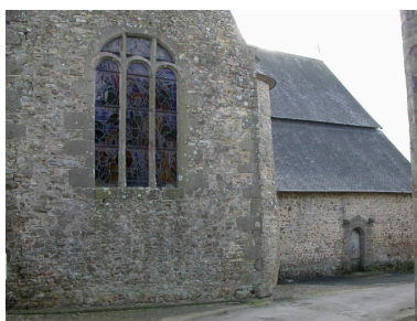
Vue nord Phot. Sabrina Dalibard IVR53_20053506207NUCA
