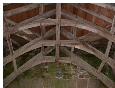
Charpente du porche Phot. Sabrina Dalibard IVR53_20053506211NUCA
