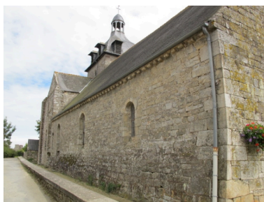
Façade nord Phot. Sabrina Dalibard IVR53_20113506613NUCA
