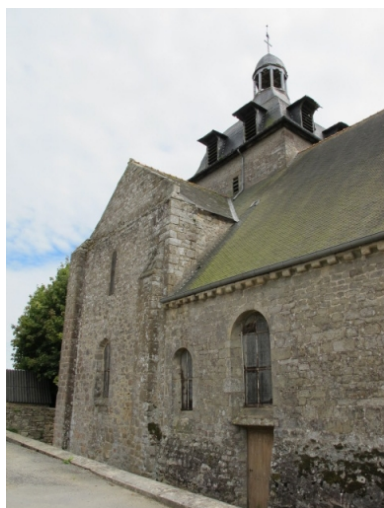
Façade nord Phot. Sabrina Dalibard IVR53_20113506612NUCA
