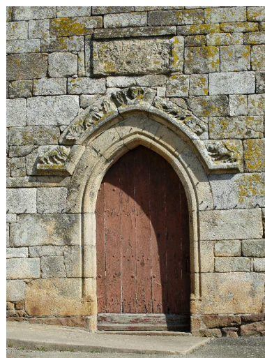
Porte ouest Phot. Norbert Lambart IVR53_20123500337NUCA
