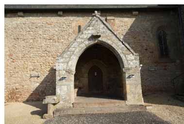
Porche sud Phot. Norbert Lambart IVR53_20123500453NUCA
