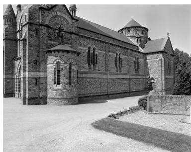
Elévation sud-est. Phot. Guy Artur, Phot. Norbert Lambart IVR53_19803500493X
