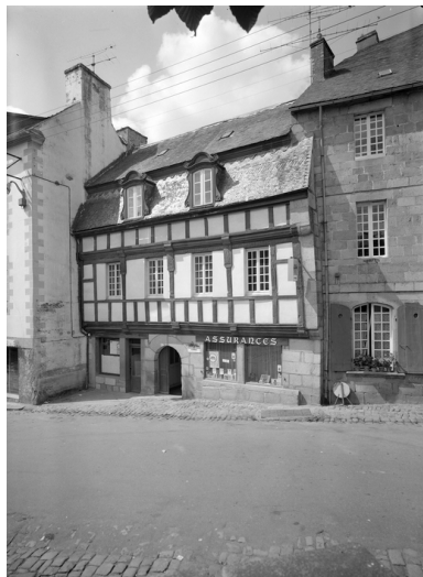
Façade Phot. Guy Artur IVR53_19742200518V
