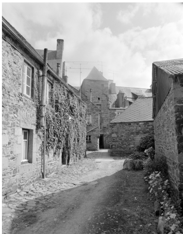
Face nord Phot. Guy Artur IVR53_19742200519X
