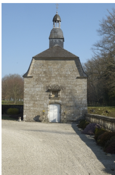
Façade principale Phot. Norbert Lambart IVR53_20113500791NUCA
