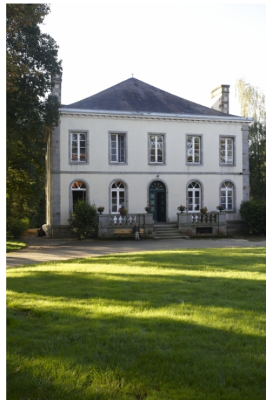
Façade principale Phot. Norbert Lambart IVR53_20113503626NUCA
