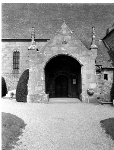
Porche sud Phot. Guy Artur, Phot. Norbert Lambart IVR53_19943500750X
