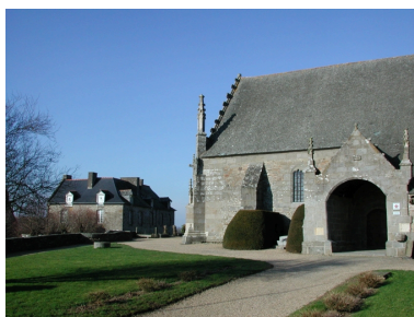
Vue partielle sud Phot. Claude Quillivic IVR53_20023506209NUCA
