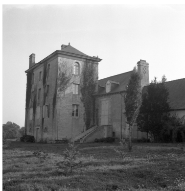
Corps de logis, vue nord est. Phot. Guy Artur IVR53_19703500822X
