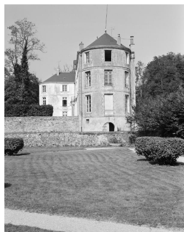
Château, élévation sud. Phot. Guy Artur, Phot. Norbert Lambart IVR53_19885601307X
