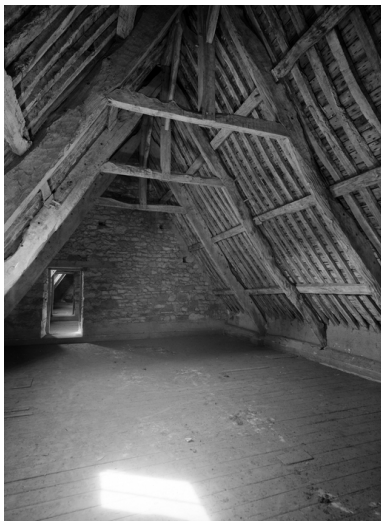
Charpente Phot. Guy Artur IVR53_19742200695V
