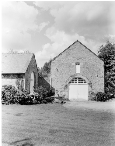
Grange 2, pignon est. Phot. Bernard Bègne IVR53_19975600630X
