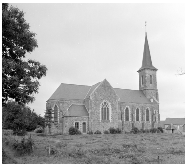
Élévation est. Phot. Jean-Pierre Ducouret IVR53_19803500570X
