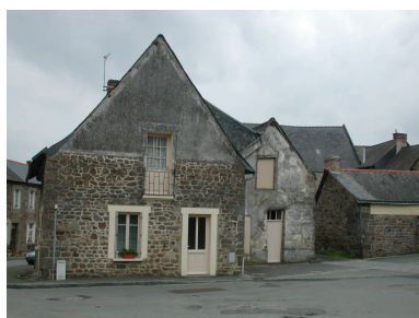
Elévation ouest Phot. Elise Lauranceau IVR53_20063511950NUCA
