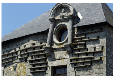
Elévation sud : lucarne Phot. Guy Artur, Phot. Norbert Lambart IVR53_19915600221ZA
