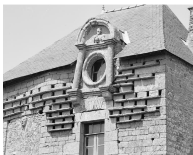
Manoir, élévation sud, lucarne. Phot. Guy Artur, Phot. Norbert Lambart IVR53_19915600216X
