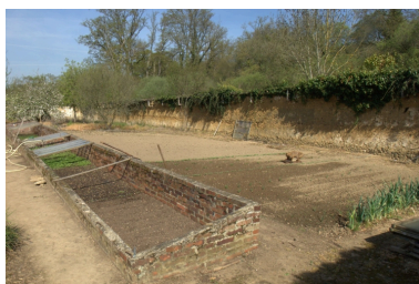
Jardin potager, serres quadrangulaires Phot. Norbert Lambart IVR53_20102202762NUCA
