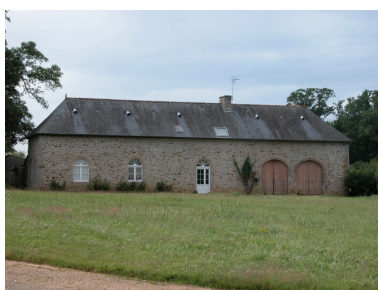
Communs, aile ouest Phot. Véronique Orain IVR53_20092210857NUCA
