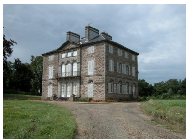
Château, façade sud Phot. Véronique Orain IVR53_20092210859NUCA
