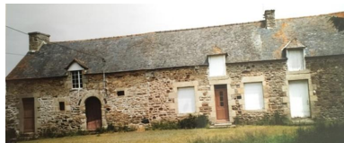
Longère de Saint-Maleu IVR53_20202208171NUCA
